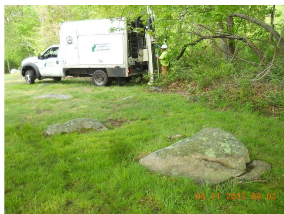
Advancement of soil boring at Black Hall site.
