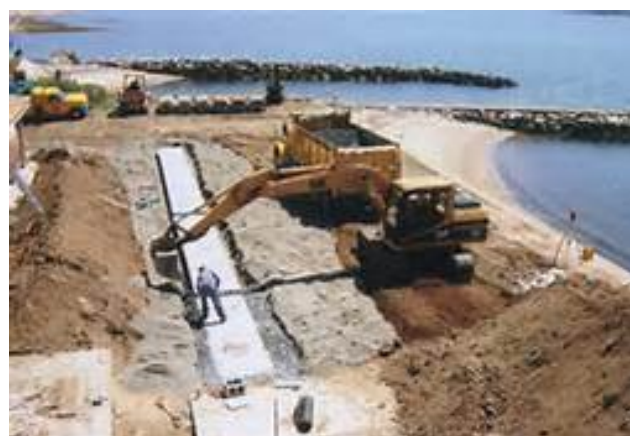
Example of on-site sub-surface disposal system construction in coastal community.
