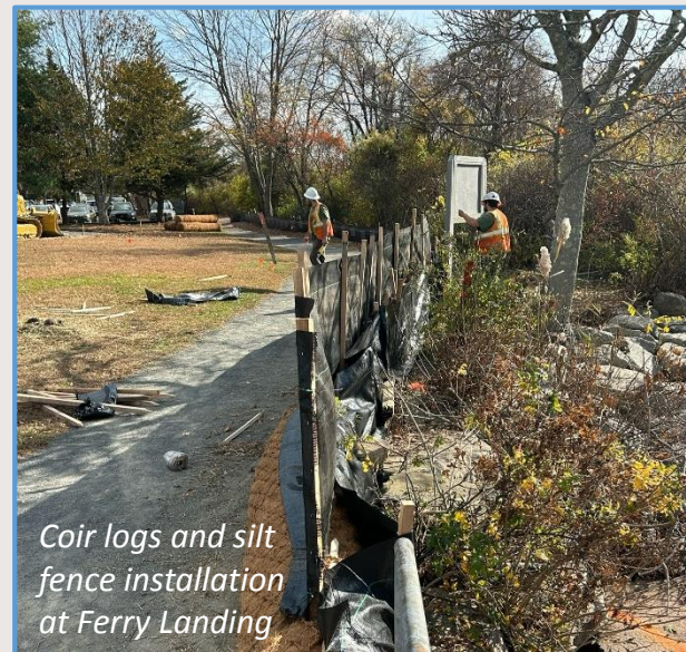
Mulch for erosion control
